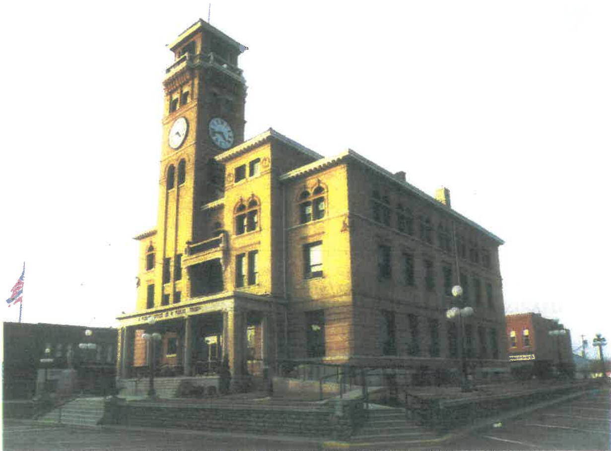
Cass County Courthouse, Harrisonville, Missouri – built in 1897
